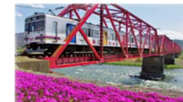
Ueda Electric Railway Bessho Line
